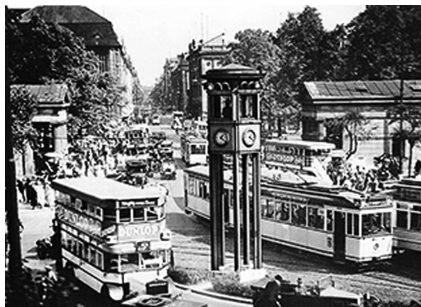
图 1 1924 年德国柏林坡茨坦广场的五边交通灯塔 Fig. 1 The famous five-sided traffic light tower installed at Berlin's Potsdamer Platz in 1924
